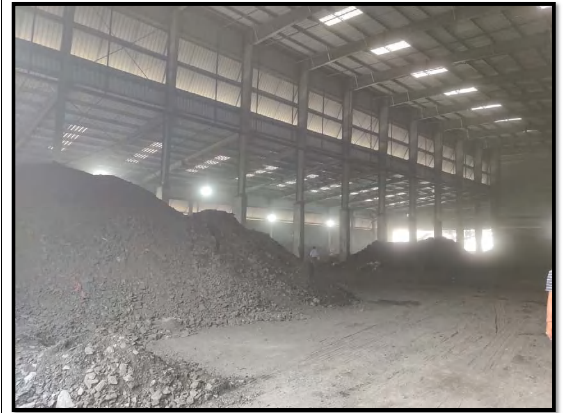
Boiler Fuel Yard
